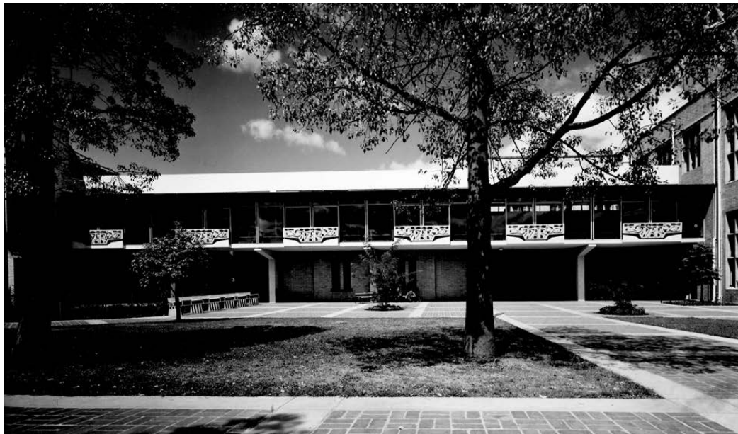
Fig. 2. Teisutis Zikaras, Relief panels for Union House , 1958. Eight form-cast concrete panels, each 2.0 x 3.0 m approximately, Parkville, Victoria, University of Melbourne, Union House. (Photographer unknown, courtesy Marcus Zikaras)
