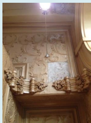
Interior ceiling tile loss
