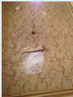
Interior ceiling tile loss
